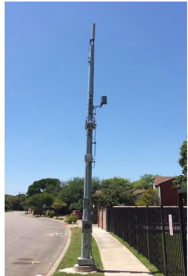
Provider Pole Installation
