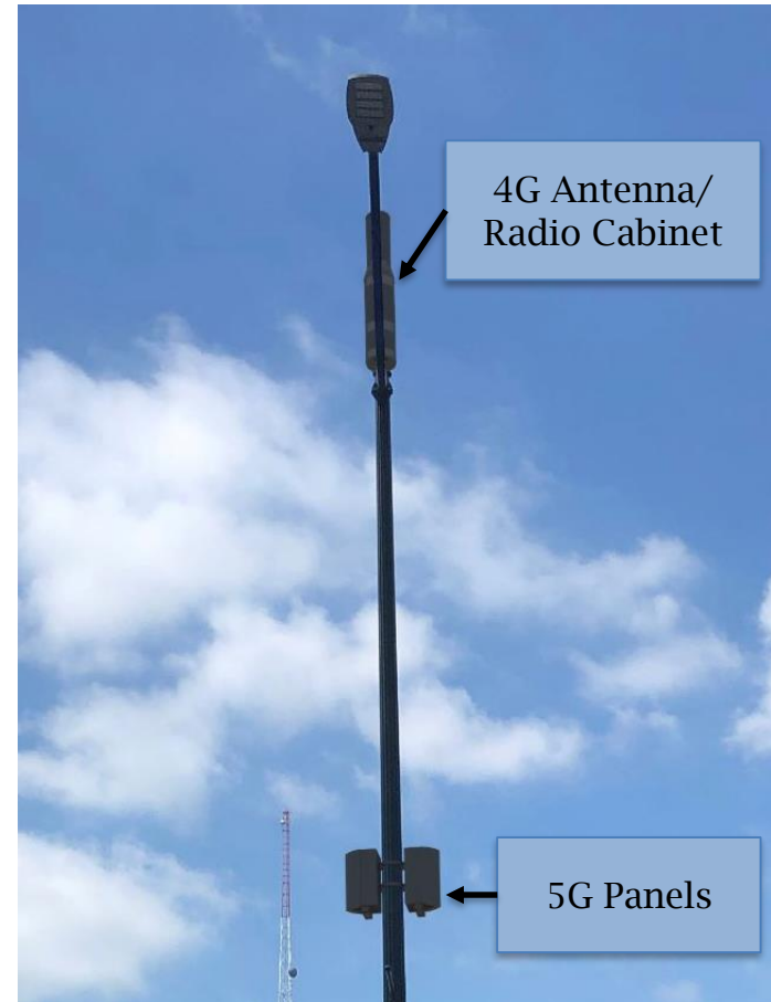
Simulation of Modified Valmont Streetlight Pole
